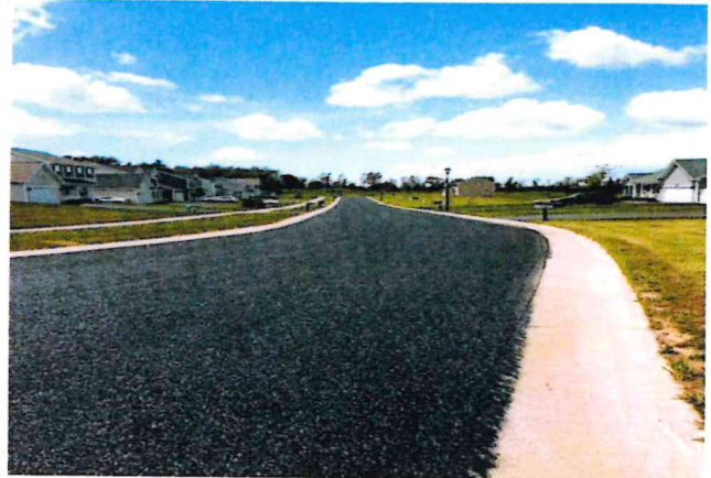
Chip Seal With Fog Seal
